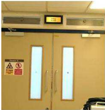
Figure 3: Illuminated Signs Displayed outside the Entrance to Theatre when X-Ray is in Use
