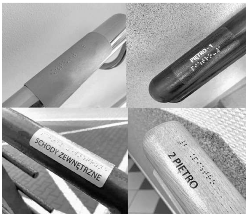
Figure 7. Prints in Braille on: aluminum overlay on the handrail, metal overlay on the external handrail, stickers on the wooden handrail
