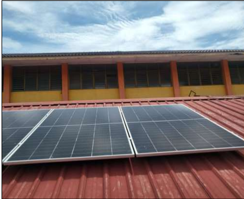
Fig 2. Six solar panels installed to generate 7,200-watt energy
