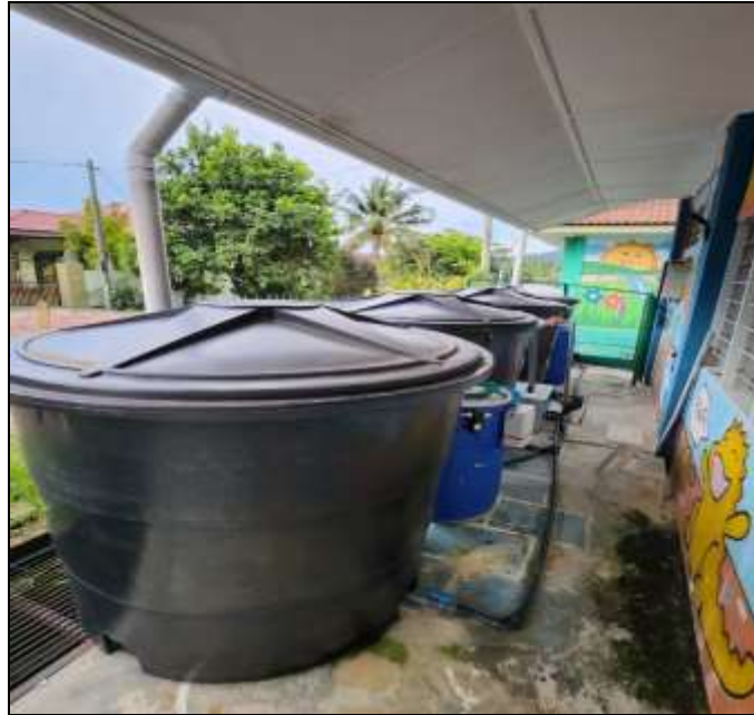
Fig 3. Four linked water tanks to harvest rain water
