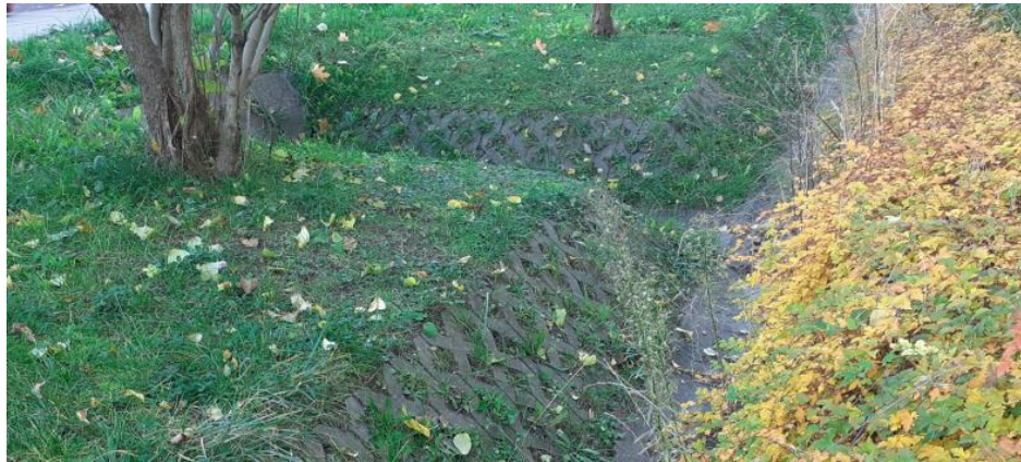
Fig 1. A part of an infiltration-drainage ditch located along a multi-family building in Częstochowa (Poland). Photo taken by the author
